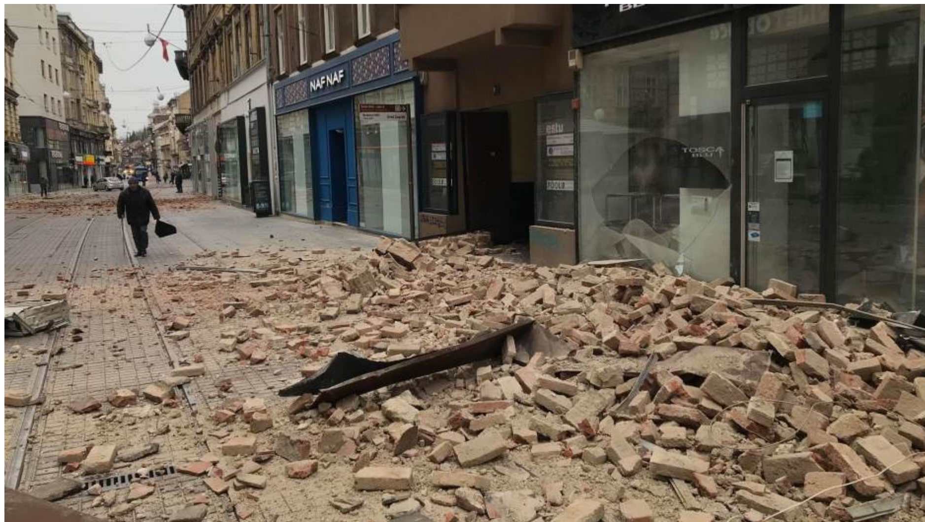
Potres u Zagrebu (foto N1)
